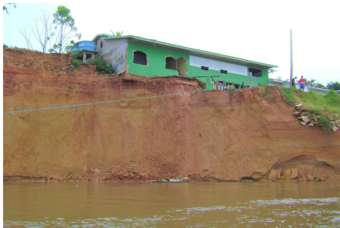
Figure 4 - Fluvial erosion on the edge of the Solimões River, city of Jutai. Photographer: Sheila Gatinho Teixeira (2010).
